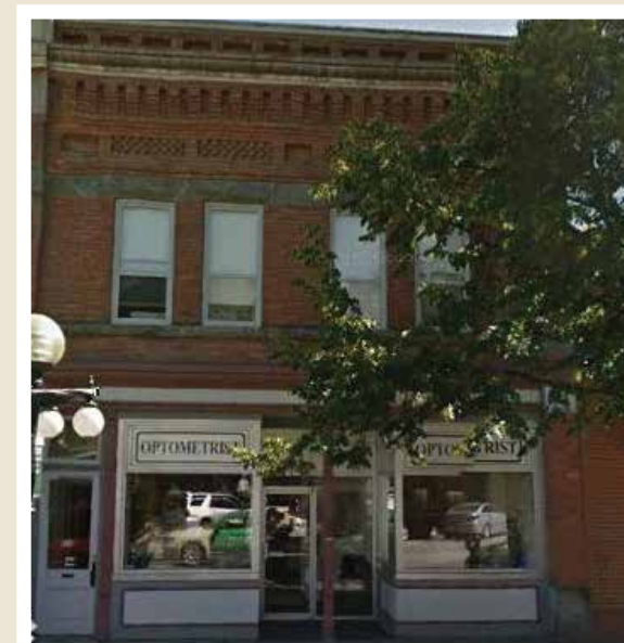
14 MCKILLOP BUILDING 364-370 Baker Street 1897 - Ewart
