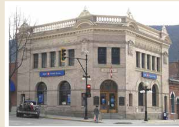
9 BANK OF MONTREAL 298 Baker Street 1899 - Rattenbury
