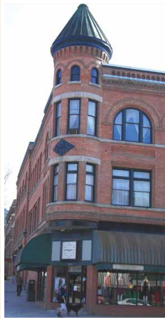
20 K.W.C. BUILDING 488-498 Baker Street 1900 - Carrie
