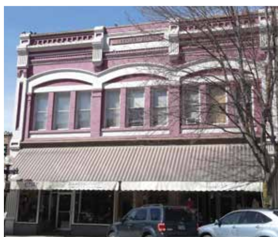
27 ABERDEEN BLOCK 571-579 Baker Street 1898
