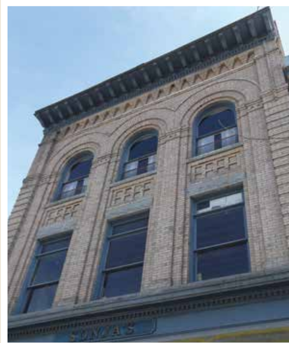
18 LAWRENCE HARDWARE STORE BUILDING 446 Baker Street 1898 - Ewart and Carrie
