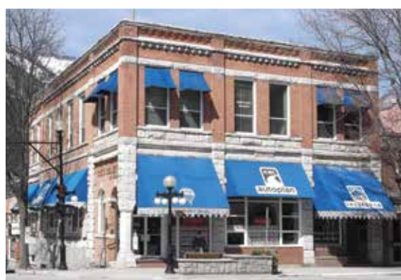
29 HOUSTON BLOCK 601-607 Baker Street 1899 - Hodgins
